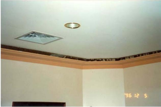
Figure 3.2: Separation of cornice from ceiling.
