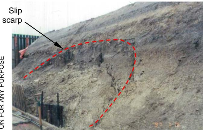
Figure 4.4.1.4: Batter failure during construction.
