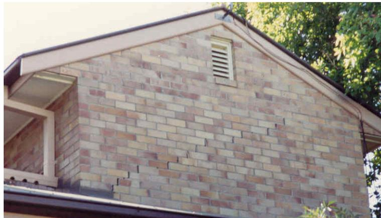
Figure 3.6: Diagonal, step-wise cracking on external brickwork of house.
