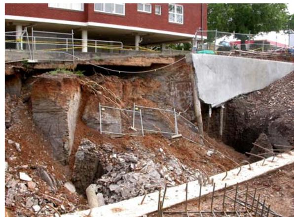
Figure 4.4.2.2: Excavation failure at Beecroft.
