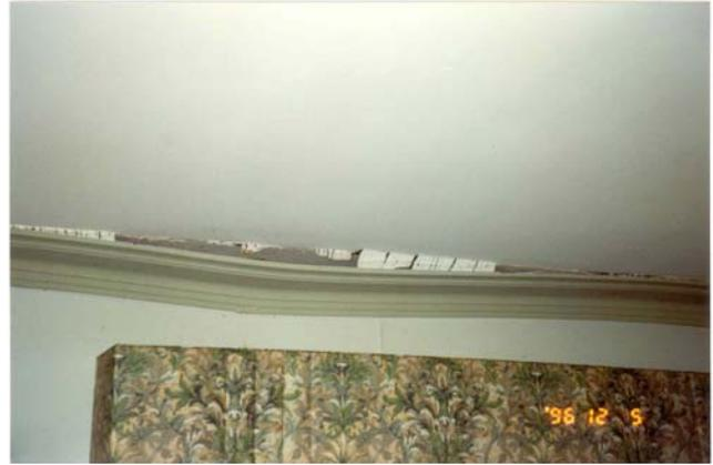
Figure 3.3: Separation of cornice from ceiling.
