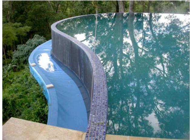
Figure 4.3.2: No 'wet-edge' due to the pool settling.
