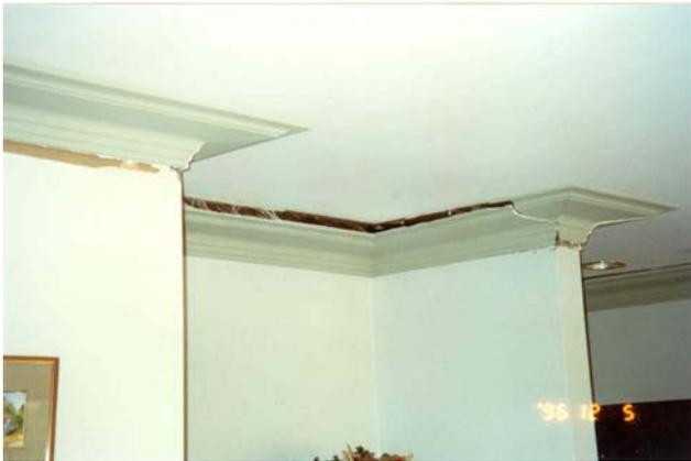
Figure 3.4: Separation of cornice from ceiling.
