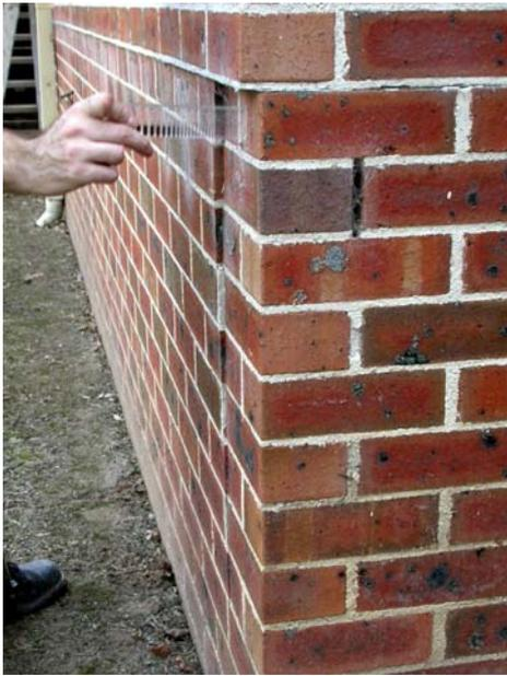
Figure 5.2.2: Horizontal separation of brickwork.
