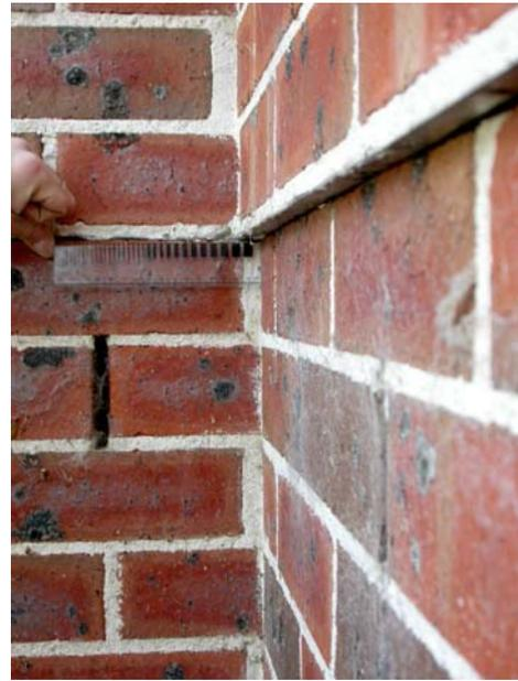
Figure 5.2.3: Horizontal separation of brickwork.
