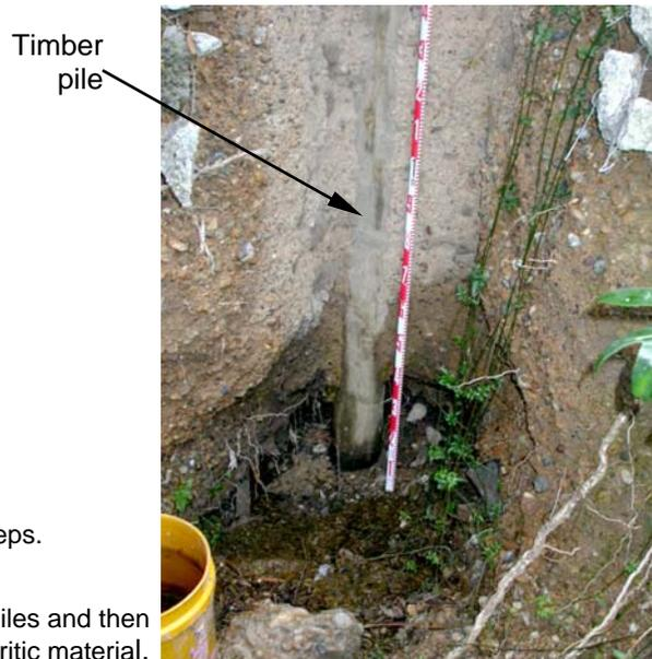
Figure 4.3.4: Timber was substituted for concrete piles and then founded on a conglomeritic material.
