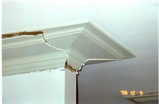
Figure 3.5: Detail of separation of cornice from ceiling.
