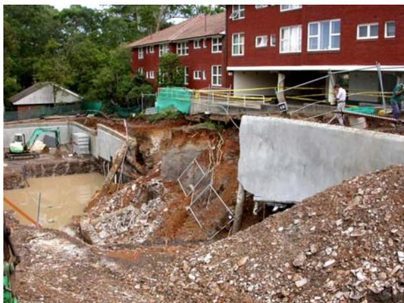
Figure 4.4.2.1: Excavation failure at Beecroft.
